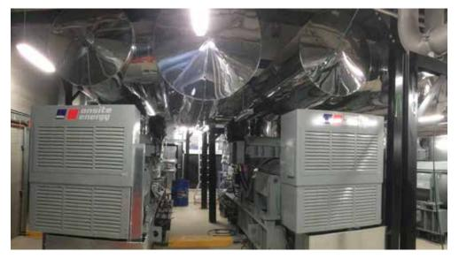
Housed within Royal Adelaide Hospital's east and west plant rooms, six MTU 20V 4000 DS 2650 diesel generators provide standby power and are capable to deliver 100 per cent capacity to the entire site in just 18 seconds.
